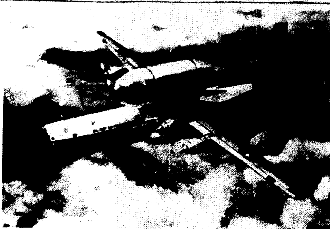
PIGGYBACK AIRLIFT —Artist's drawing shows an Air Force C-133 carrying the second stage of a Saturn C-1 missile in piggyback fashion. The method was proposed by the National Aeronautics and Space Administration to airlift the second stage from tests in Sacramento, Calif., to its launch site in Cape Canaveral, Fla., in only 10 hours. The original plan, requiring 24 days, called for shipment by barge.
