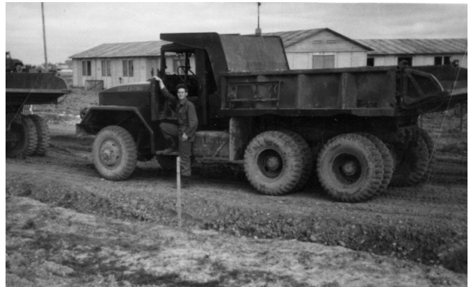
Dump Truck on Gravel Bed
